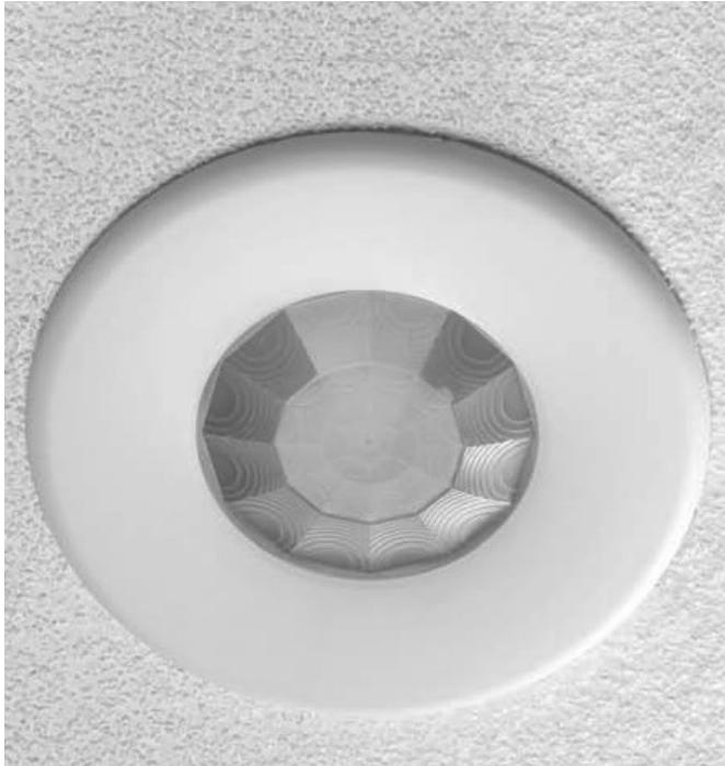
The PIR (passive infrared) presence detector provides automatic control of lighting loads with optional manual control.
