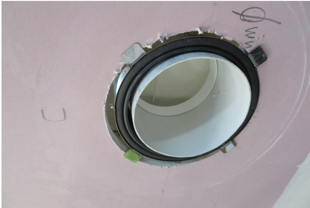
Ceiling fan cuff (125 mm) – view from unexposed face prior to the ceiling fan installation
